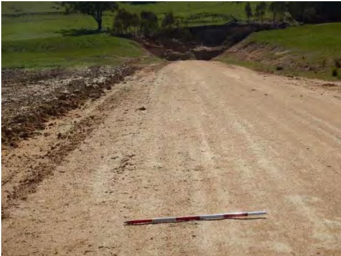
Plate 5 Visibility along vehicle access track, SU2 facing north-west (M.Aitchison 18/09/2018)
